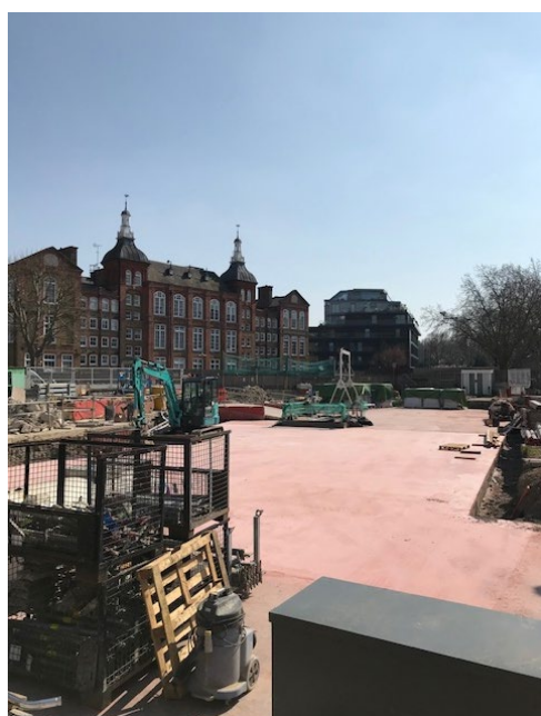
Fig. 1 Waterproofing at the NLE Kennington Green site
